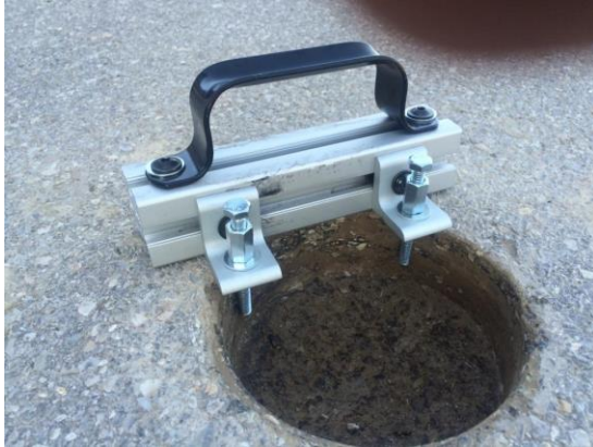
Place the Depth Guide in the core as a point of reference for proper adhesive fill Level. Proper depth of gauge is 35mm.
