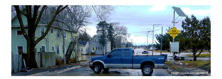
For the warning alerts, Eric and his team selected solar-powered BlinkerSigns, which are MUTCD-compliant, LED-enhanced signs created by TAPCO. They're placed on three poles ahead of the high water area so drivers have the time and space to turn around. A wall-mounted sensor detects when the water reaches a certain threshold and triggers the flashing BlinkerSigns.
