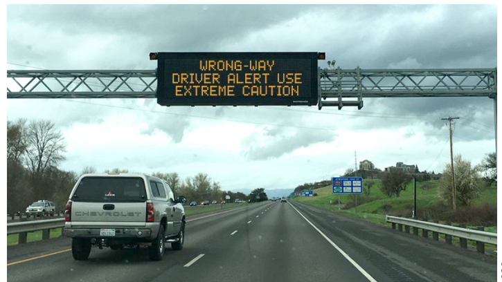
Warns drivers on system-integrated overhead dynamic message boards
