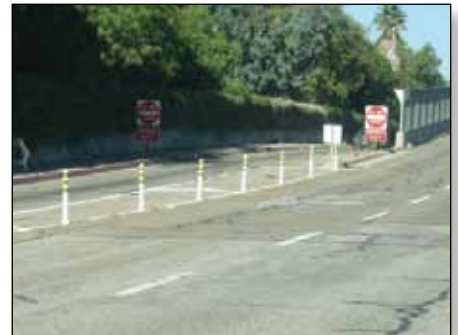
Separation of merging lanes on freeway off-ramps
