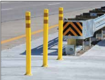
Protection of impact attenuators at frequent impact locations
