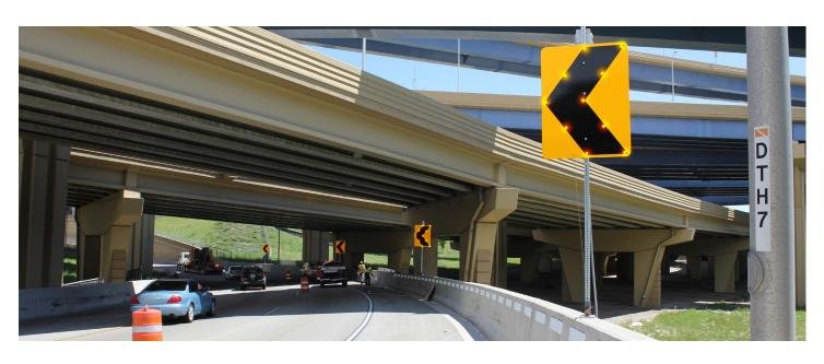
Due to the proven success of the curve warning system at that location, WisDOT installed the system with sequentially flashing signs at another one of the busiest interchanges in the state, the Zoo Interchange, when it was being completed in fall 2017. Since then, the interchange has experienced fewer collisions than the statewide average, despite the high traffic volume.
